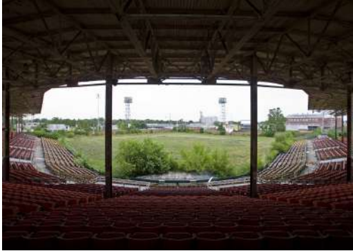
Bush stadium 2009, Indianapolis USA
