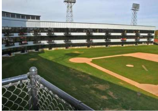
Bush Stadium stands, Indianapolis USA
