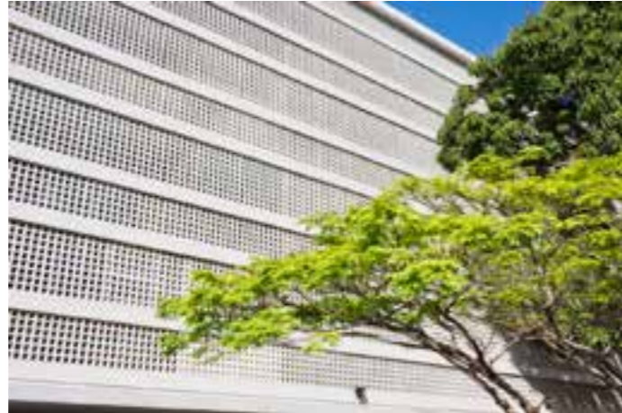
II.C.4. 4. Residential block service facade with cobogó.
