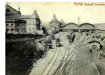
New railway station building and vaulted structure above the rails, which consumed 2,000 tons of steel, 1.2 million rivets, 18,000 m 2 of zinc sheet for roofing and over 200 pieces of large-scale glass panes. 1918 | photo: stock photos Profimedia
