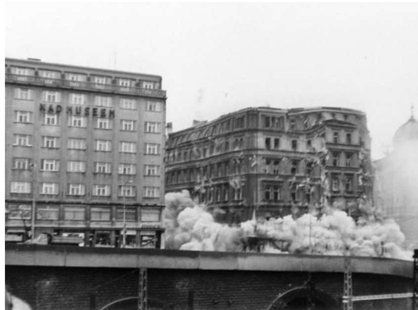
Fig. 2 Demolition of a building in Vinohradská Street during the construction of the North-South Trunk Road
