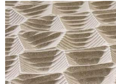
Dense gypsum fiber board panels reflect sound. Parametric design by One to One image © Johannes Ait
