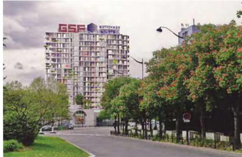
NEW ADDITION Self-supporting structure are added on the periphery of the existing building at every floor, to extend the living rooms, create closeable terraces and balconies
