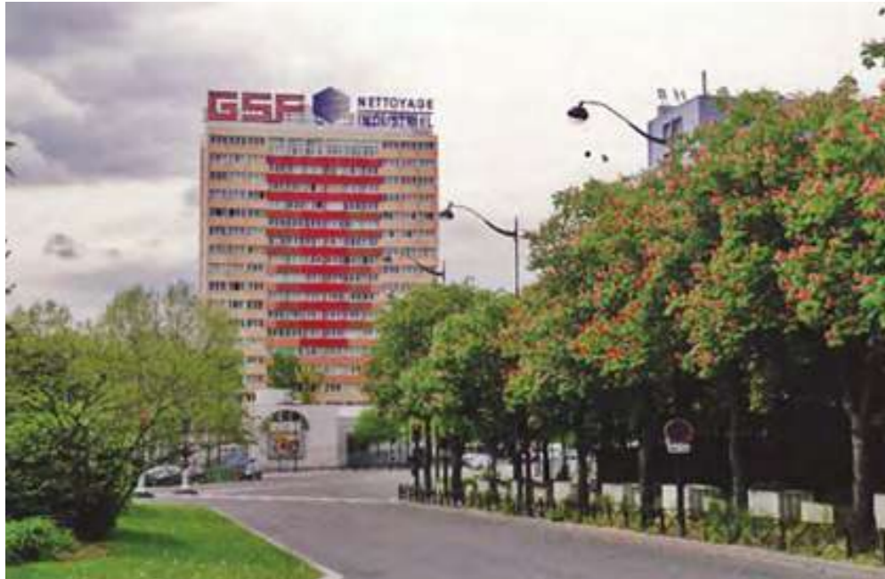
ORIGINAL BUILDING This high rise block of 16 storeys includes 96 apartments
