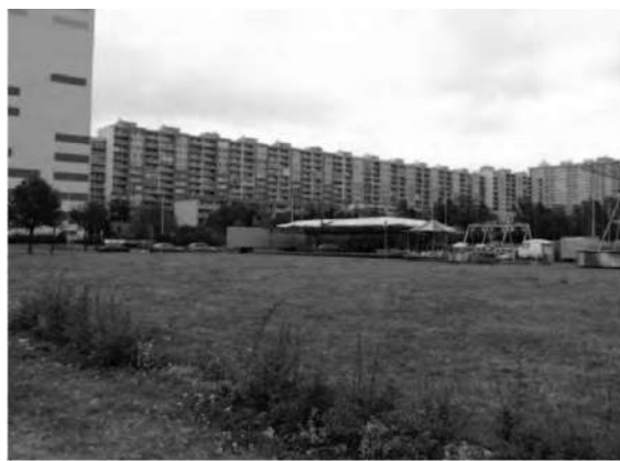
■ prefabricated houses with a length of about 250 m
