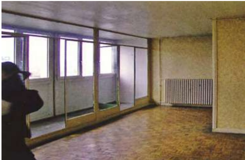
ORIGINAL APARTMENTS The existing facades with small windows were removed
