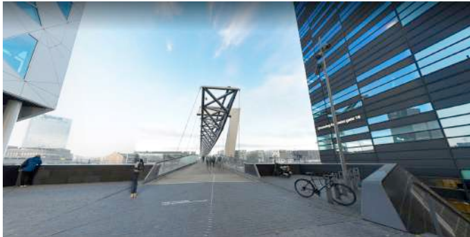
OSLO, NORWAY. PEDESTRIAN BRIDGE.
