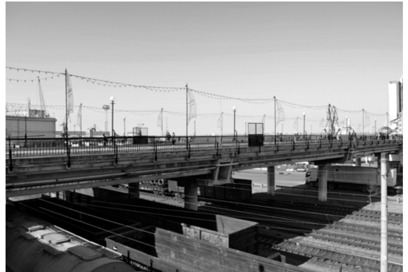
Bridge Structure Across Railways
