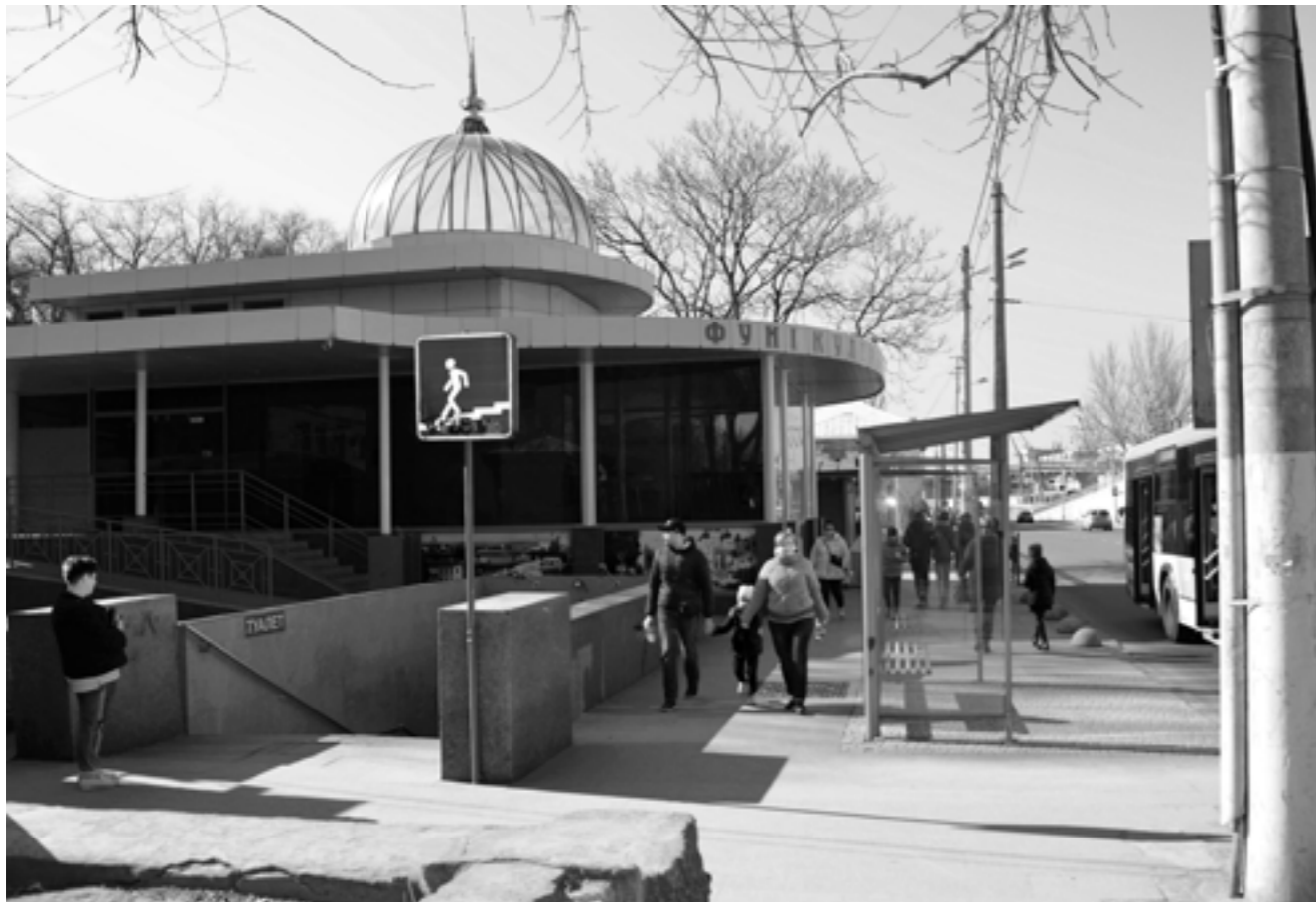
Entrance to the Funicular/Entrance to the Underpass
