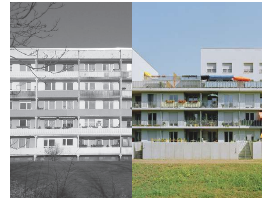
Downsizing of a panel building. Source: archdaily.com
