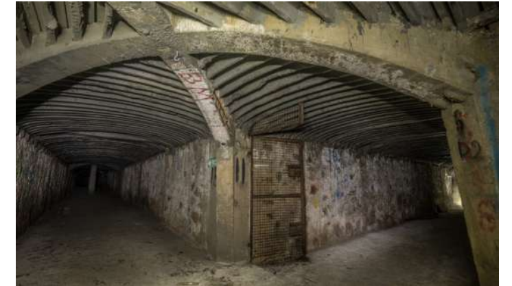
The ceiling of the air-raid shelter is in a strip-shaped arch, with a distinct European style
