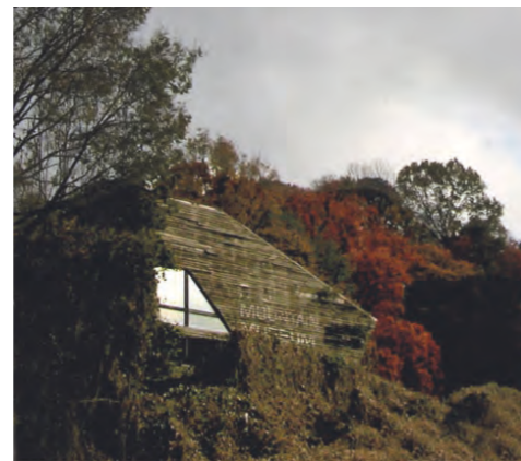
Red Mountain Museum before demolition
