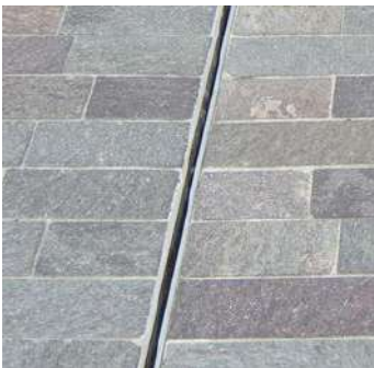
Paving 17- Drainage line- Zinc coated steel
