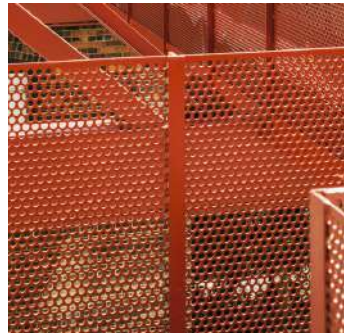
22 Red line-perforated steel grate. Walkway material, light structure.
