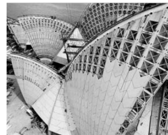
The simple sphere geometry and the construction of the shells
